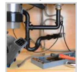
Works in Tight Spaces for Tough Drying Jobs
